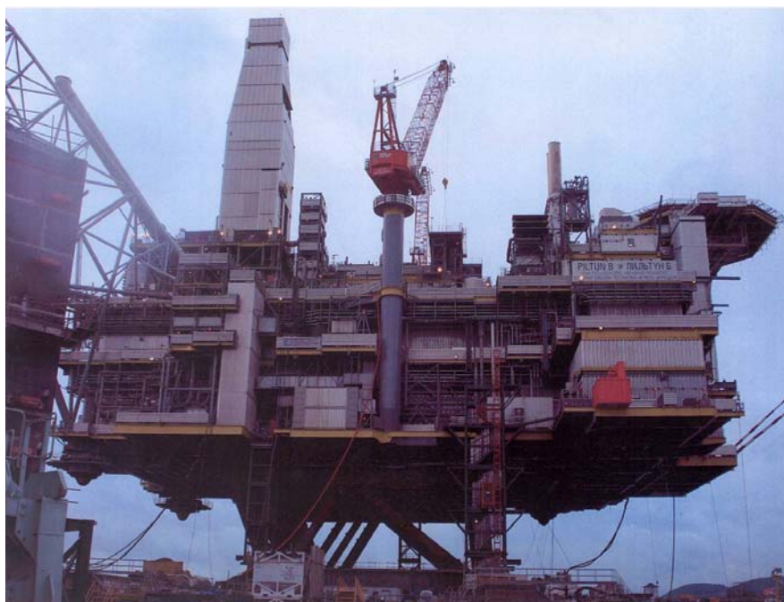
Fig. 1 The world's biggest offshore platform having a daily capacity of 2.6 M m 3 gas and 70 000 barrels of oil
