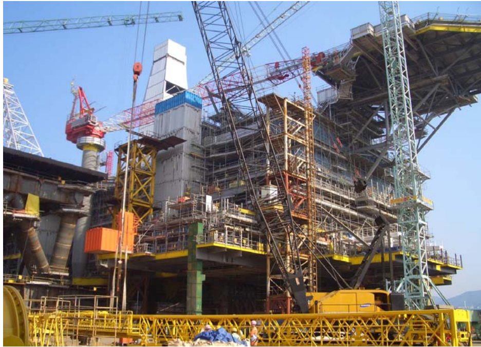
Fig.2 The dimensions of the platform is approximately 95 m x 130 m x 120 m
